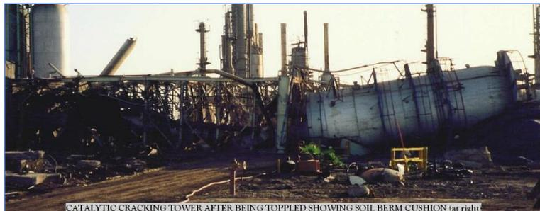
CATALYTIC CRACKING TOWER AFTER BEING TOPPLED SHOWING SOIL BERM CUSHION (at right)
